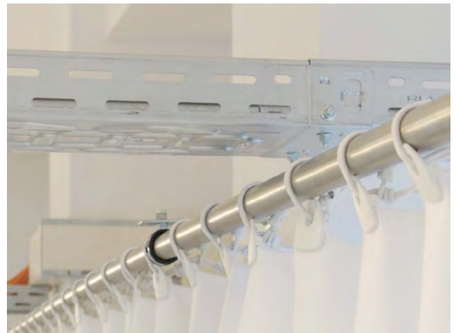
Acoustic curtains in white stage molton absorb sound. (Photo: Fabian Scholz | Image Knowledge Gestaltung 2015)
